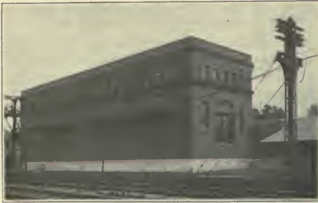
FIG. 495. SUBSTATIONS. Exterior View of Substation of the New York Central & Hudson River Railroad. The Building is Constructed of Brick and the Transmission and Feeder Supports are of Structural Steel.
